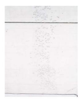
Spalling in a line, as shown in this photo, occurs when salt is brought onto your driveway with your car's tires. This can also happen when snow is not shoveled, but is driven on and allowed to remain as ice tracks on your driveway.
